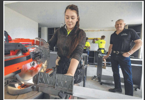
Hamah Mottram works with a saw at a Waterloo site on Tuesday as Perth-based construction company owner Robert Shaw looks on. OLIVIA MORTY
